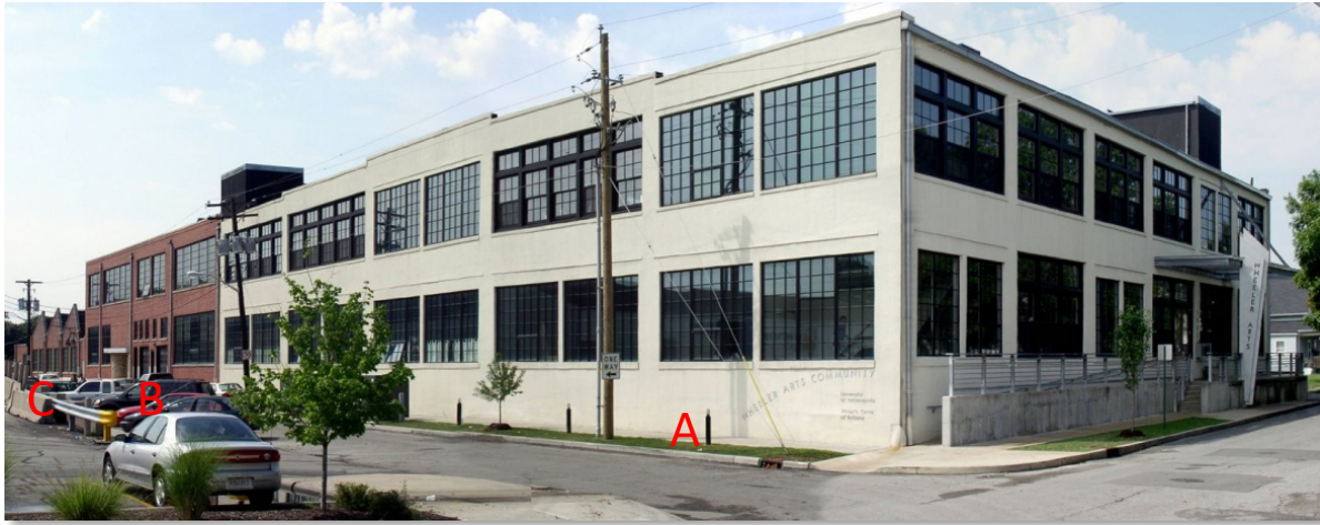
Wheeler Building Exterior
